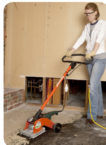
FCS10 Removing VCT from concrete.
